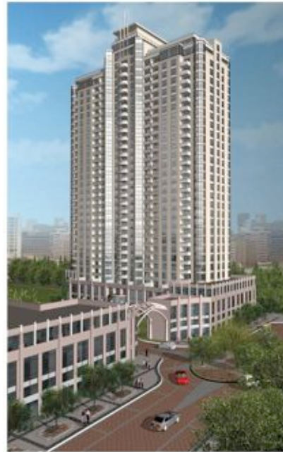
GRAND TRIOMPHE II (LEED-NC Candidate) 34% Energy Savings
